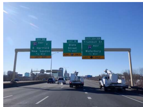
Figure 1. Sign support 21311 on I-84, Hartford, Connecticut
