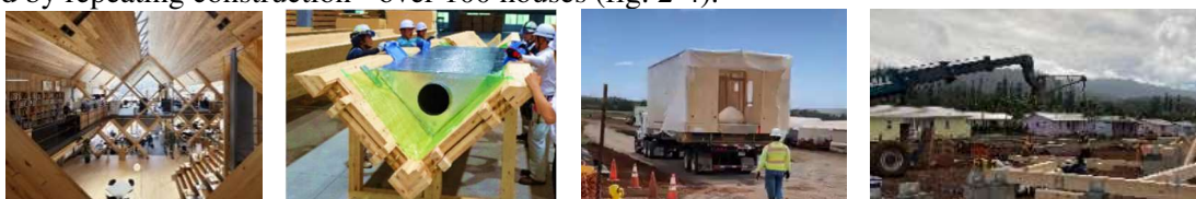
Figure 2. 1)interior view, 2)duct in CLT beam, 3)test unit delivery, 4)housing construction site
