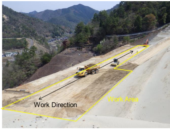
(a) Embankment site
