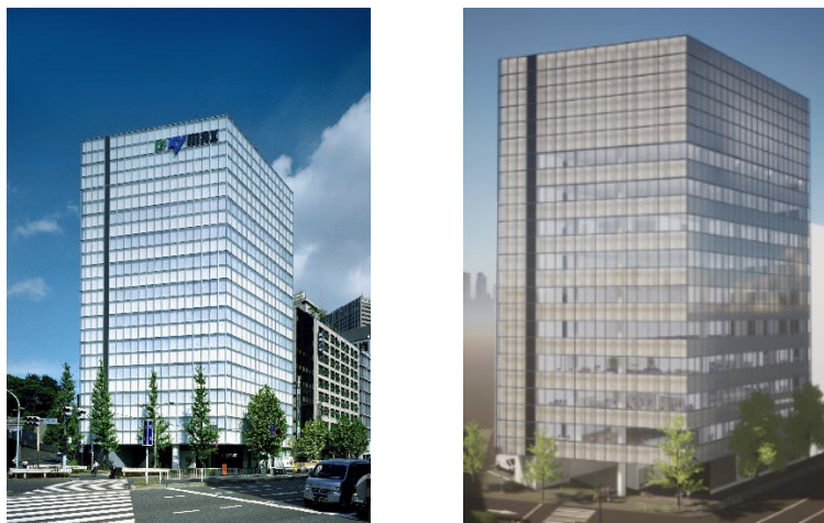
Figure 2: Comparison between the actual building (left) and the rendered BIM model (right)
