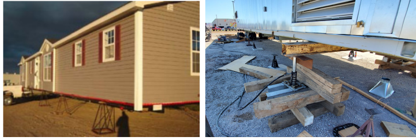
Figure 1. Module Lifting via Hydraulic Jacks: Mini-Home (left)[3], Mojave Bloom (right)
