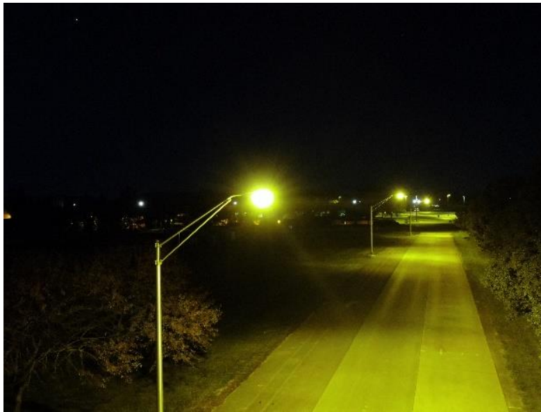
Figure 2. INDOT roadway lighting test facility
