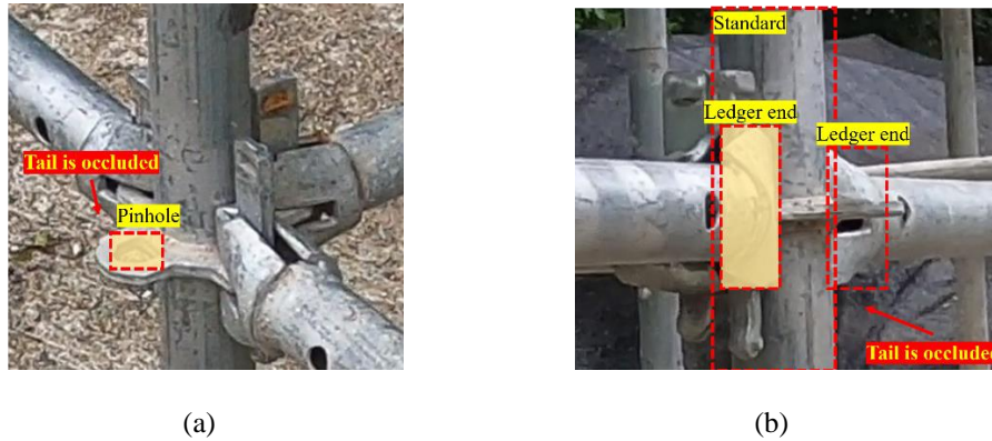
Figure 3. Examples of poor quality joint images; (a) vertically angled, (b) horizontally angled
