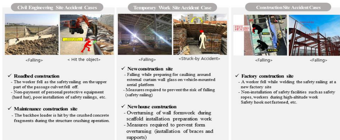
Figure 12. A case of safety accident in civil and building construction
