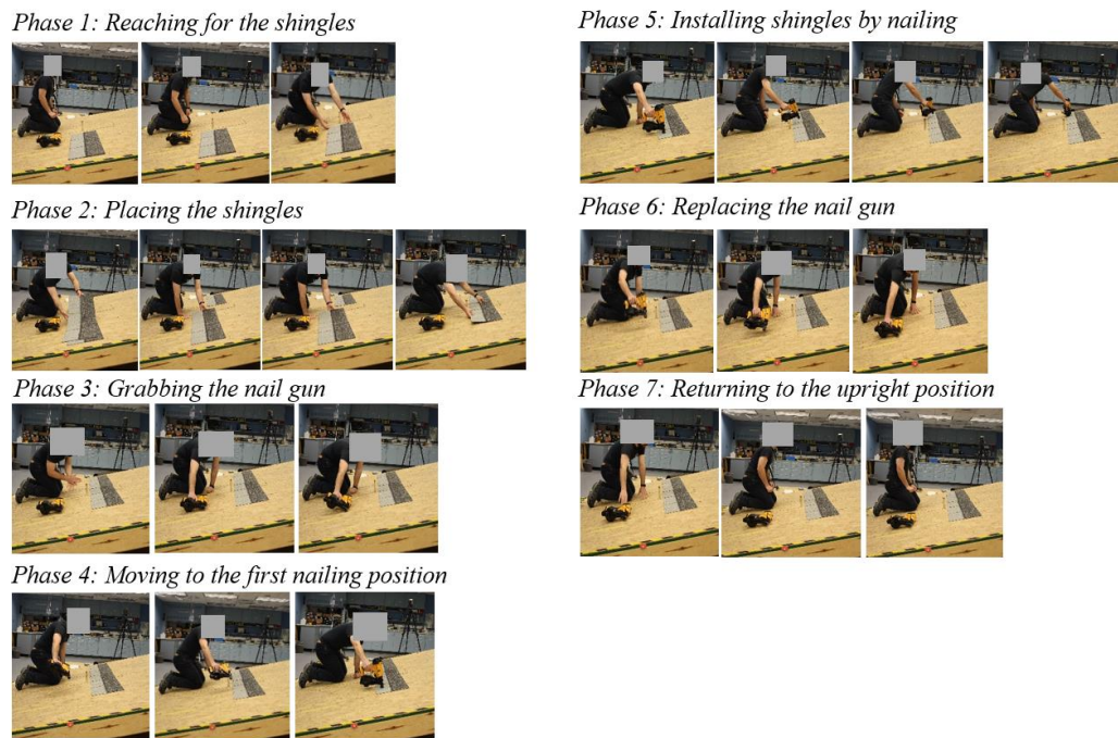
Figure 3. Seven phases of shingle installation process
