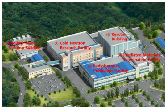
Fig. 2. Decommissioning Sequence for the Research Reactor and Related Facilities.
