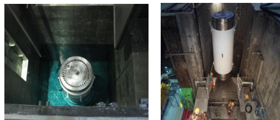
Fig. 1. Cask transportation w/o lid bolt fastening (Loading pit -> Decon. pit).
