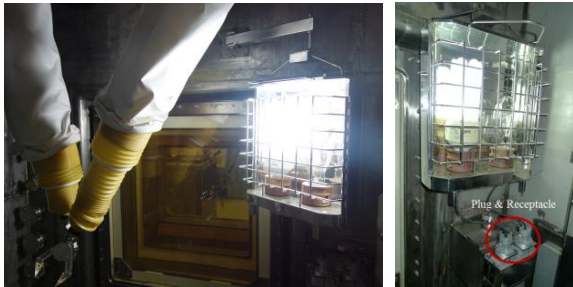
Fig. 4. Cell lighting device installed in the argon cell.
