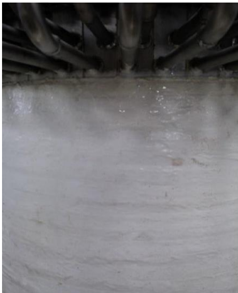
Fig. 1. Photo of external wall coating material of melter.
