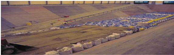
Fig. 5. Waste Placement in Trench at Morvilliers.
