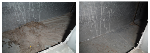
Fig. 4. Photos before and after duct cleaning.
