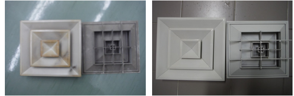
Fig. 1. Photos of diffuser before and after cleaning.
