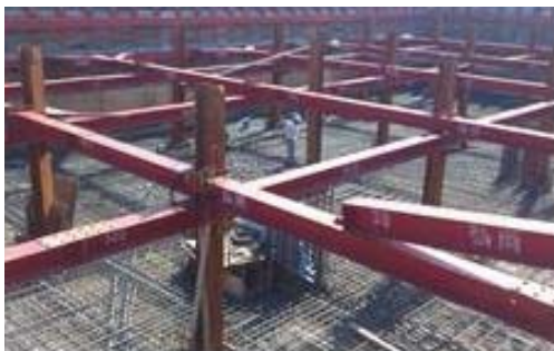
FIGURE 2 CONSTRUCTION OF B2F
