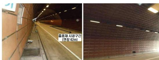
Fig.4 Absorbing material installed in Tunnel-D
