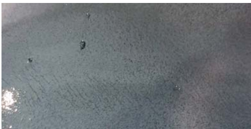
Fig. 4 Crack initialed at the surface of test wheels
