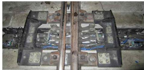
Fig. 1 Installation of contact detector
