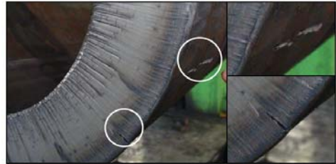
Fig. 04 Result of jack-up leg chord bending test
