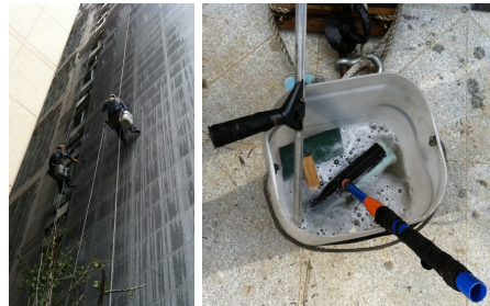
Fig. 1 Conventional cleaning work and tools
