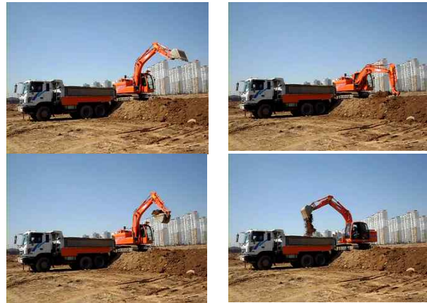
Figure 6. Excavation and Loading of IES
