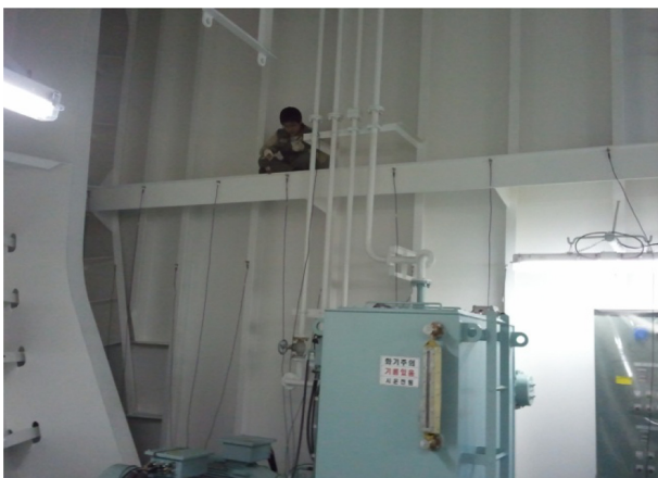
Fig. 10 The picture of the fresh water tank (F.W.T.)
