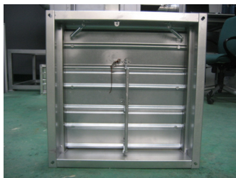
(a) Fusible link and spring side
