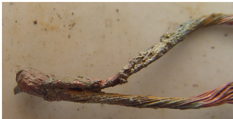
Figure 2. Fire melting damage
