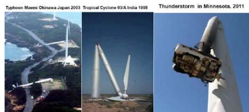
Fig. 1. Buckled steel wind power tower
