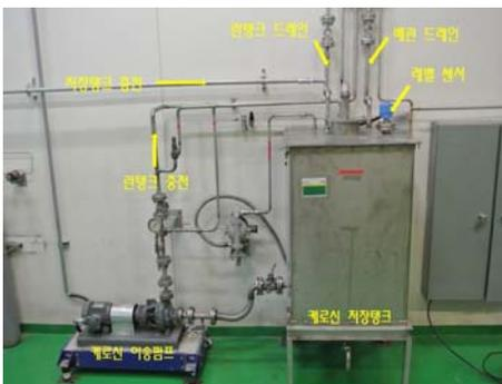
Fig. 4 Kerosene Storage Tank
