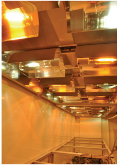
Fig. 3. Light source system of walk-in growth chamber
