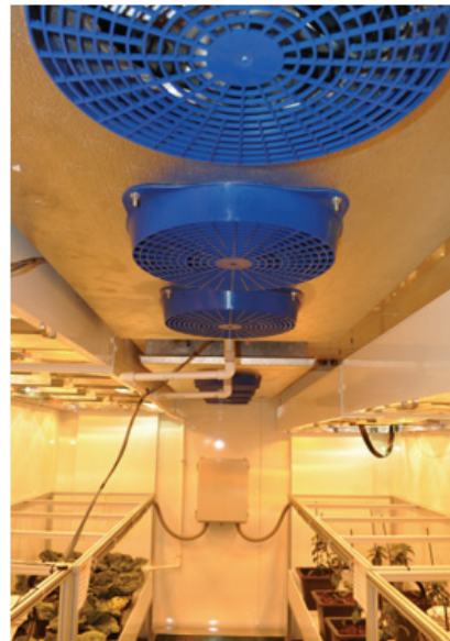
Fig. 4. Forced convection system of walk-in growth chamber
