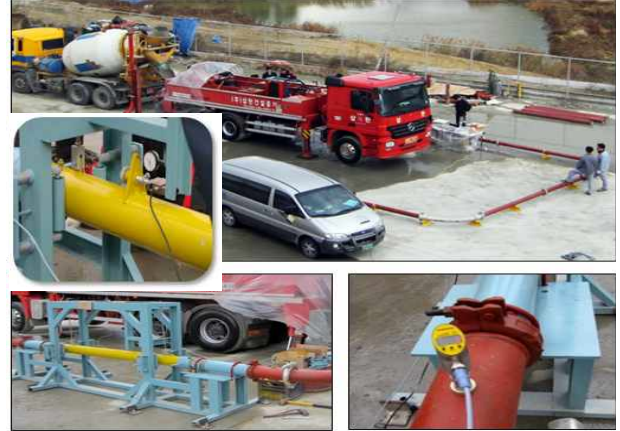
Figure 2. Pumping test for concrete
