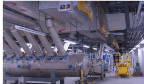
Fig. 7. Argon system and duct line of PRIDE.
