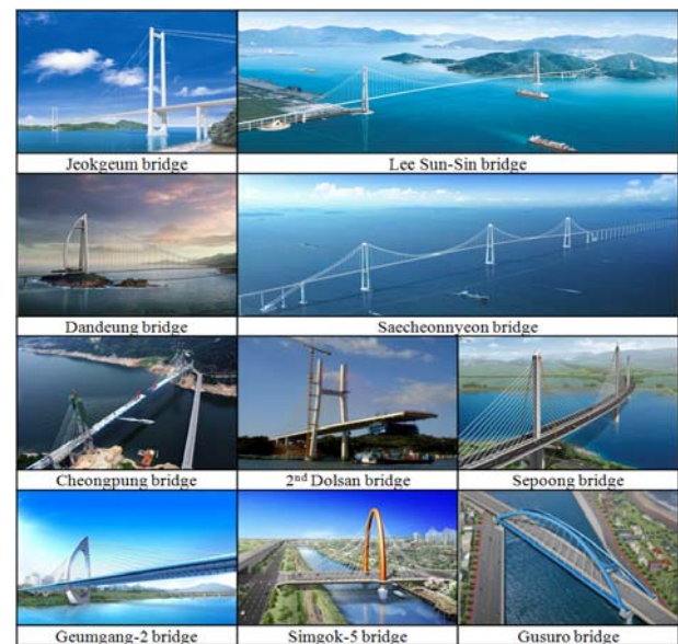
Figure 2. Long span bridge in Korea(under construction)
