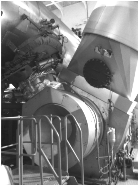
Fig. 3 Installation of swing gate valve onboard a vessel
