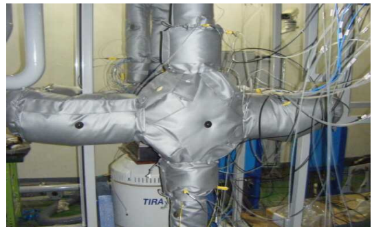
Fig. 9 Performance Test Setup with Insulation
