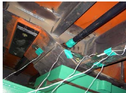
Fig. 3 Strain gauge of the underframe
