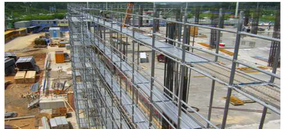
Fig.2 Scaffolding on construction site installation form
