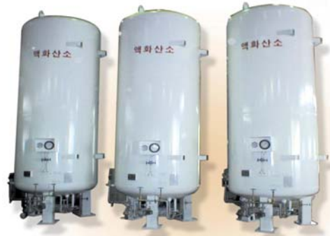
Fig. 1 Analog measurement of level of very low temperature liquefied gas
