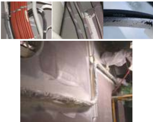
Fig. 1 Coating stains on electric cable sheath(above) and protection by vinyl material(below)
