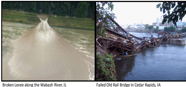
Figure 3: Midwest Floods and Infrastructure Failure (2008)
