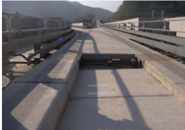
Fig. 4 Road Surface and Guide Rail
