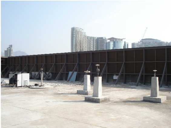
Figure 5. Deformation monitoring test site
