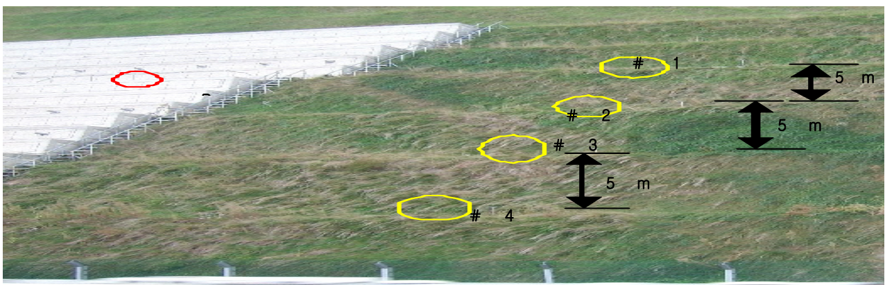
Figure 9. The roadside slope and the points monitored
