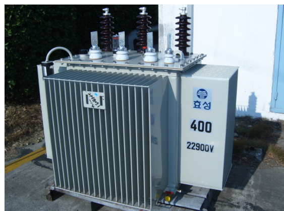
Fig.1 400kVA 22.9kV Distribution transformer (Hyosung)
