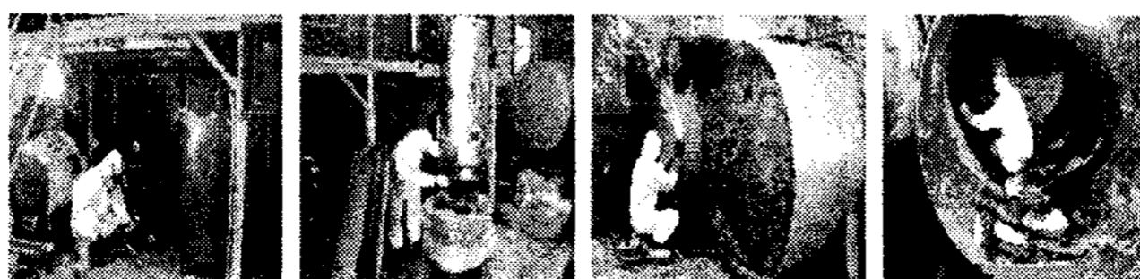
Fig. 1. The decommissioning process of the liquid waste treatment facilities.
