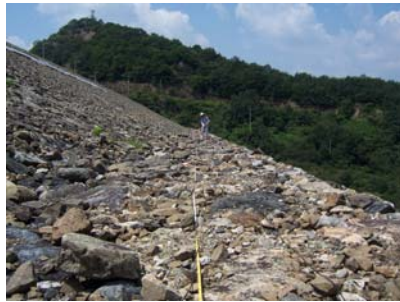
(a) survey line on berm
