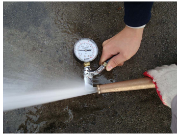
Fig. 3 Test of discharge pressure in indoor hydrant system
