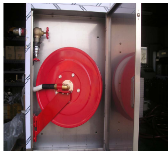
Fig. 2 Hose reel hydrant system
