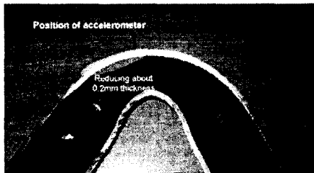
Fig. 14 Picture of test pipe section
