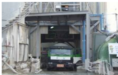
Loading a concrete batch
