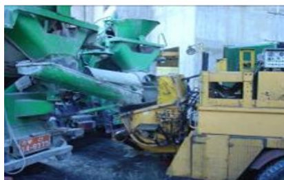
Concrete pouring at the site
