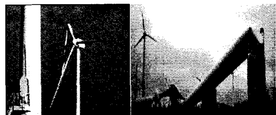
(a)Blades fracture (b)Support bending
