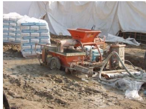
Fig. 6 Injection of cement grout.
