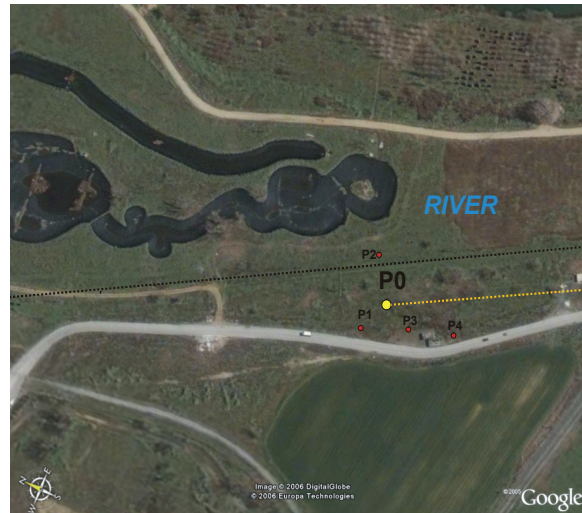
Fig 2. The water injection installation with injection and monitoring wells (P0, P1-4).
