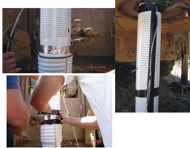
Fig. 3. Photographs showing the ERT cable installation.
