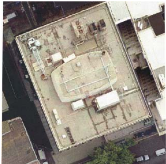
Figure 2. Building roof top has been ortho-rectified although small roof top structures have not.
